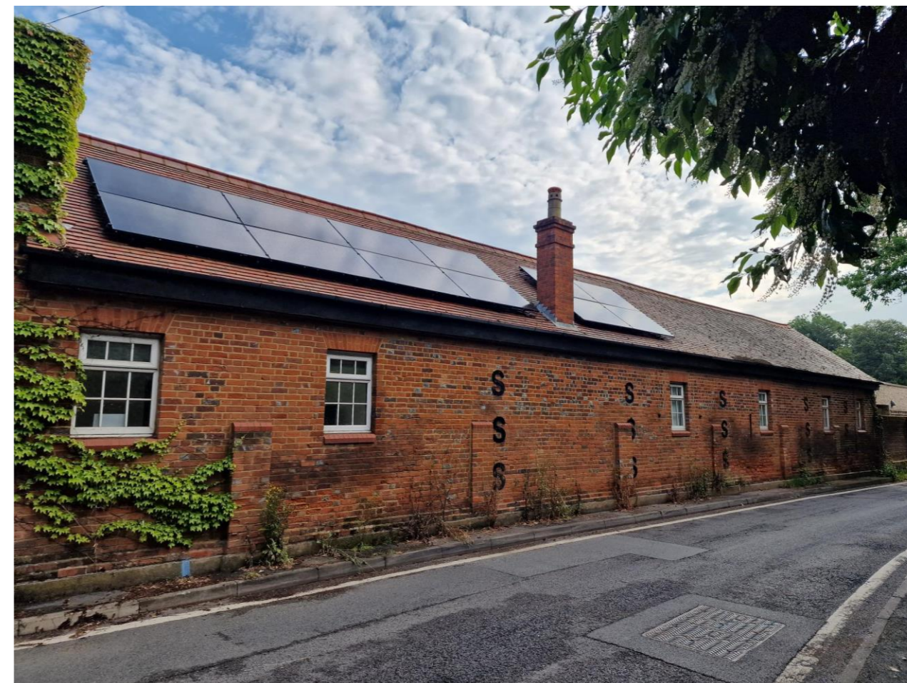
PV panels on Braywick Nature Centre
